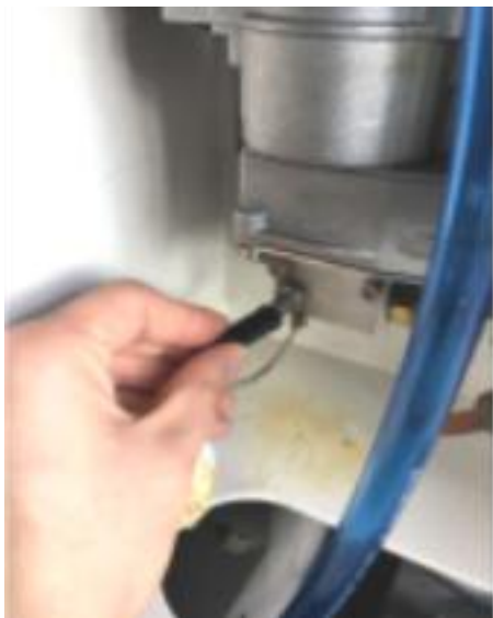
盖好润滑泵注油口盖
